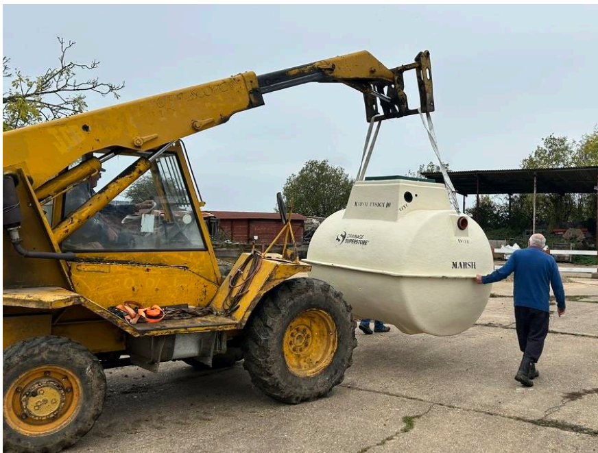
New sewage treatment plant arriving at Ray Beales barn
